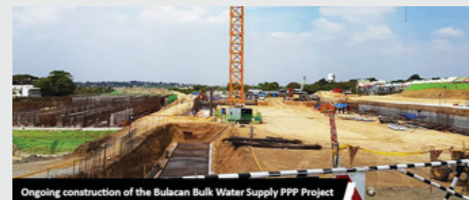
Ongoing construction of the Bulacan Bulk Water Supply PPP Project
