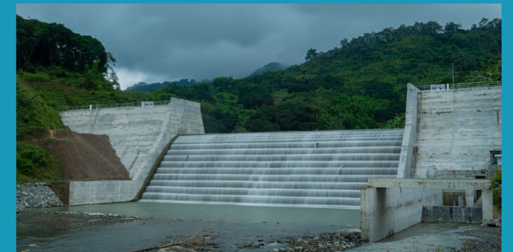
Phase 1 of the Wawa Bulk Water Supply Project started commercial operations in October 2022. It supplies the initial 80 million liters per day of raw water.
